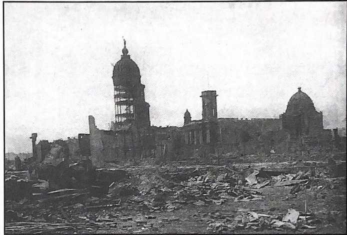
City Hall Tower, after the San Francisco earthquake
